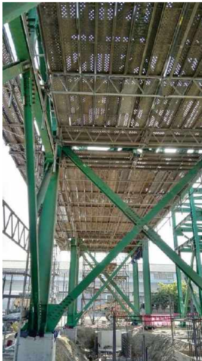
Work: Talara / Interconnections rack
