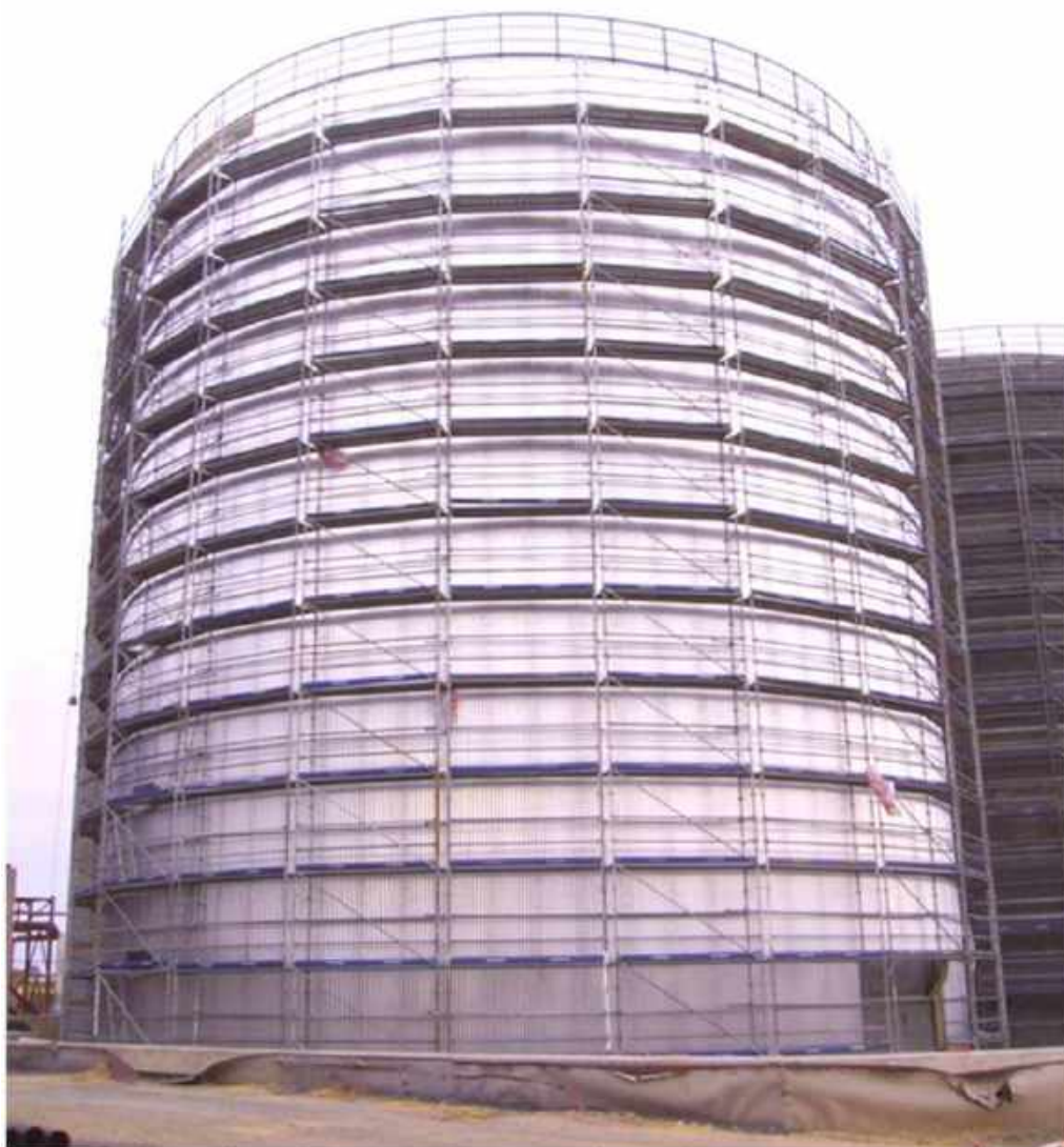
Work: Tank in BioOils plant
