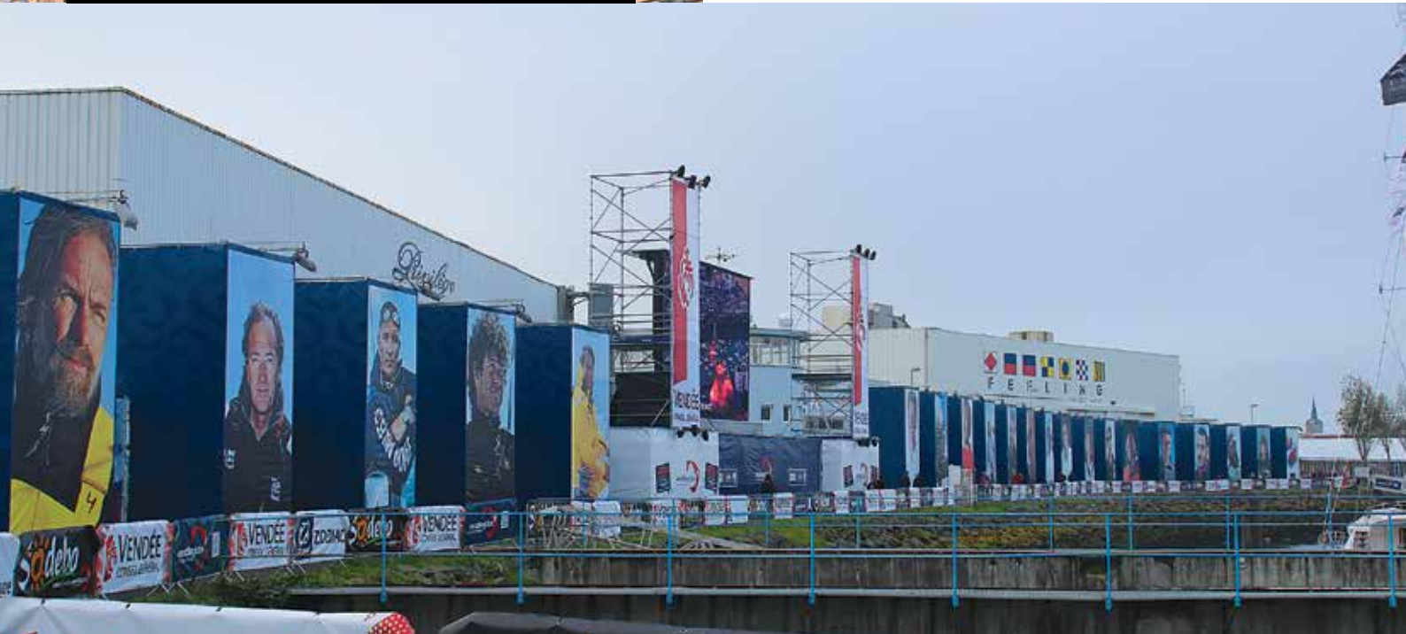
Les Sables-d'Olonne, Vendée Globe race: 180 m long scaffolding wall consisting of "totem towers" supporting the sailor's portraits.
