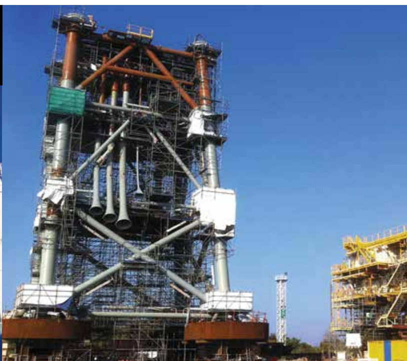
Fos-sur-Mer: scaffolding for the construction of modules for the "Anguille" offshore platform.
