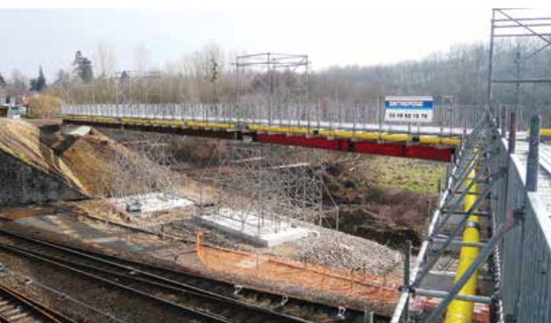
RN 21, between Limoges and Périgueux: temporary footbridge during reconstruction of the bridge over the railway.
