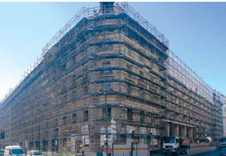
Paris, Louvre post office: 230 tonnes of Multicrab scaffolding for the 9200 m 2 of the building's four sides.
