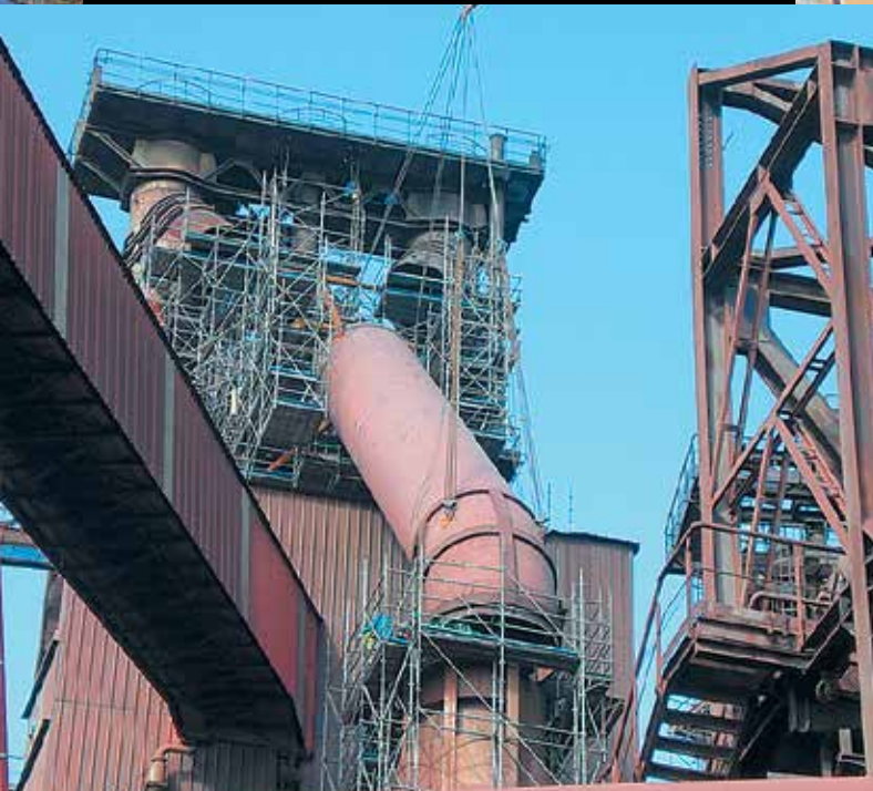
Arcelor Mittal Atlantique et Lorraine site: scaffolding for maintenance work on blast furnace No. 2.
