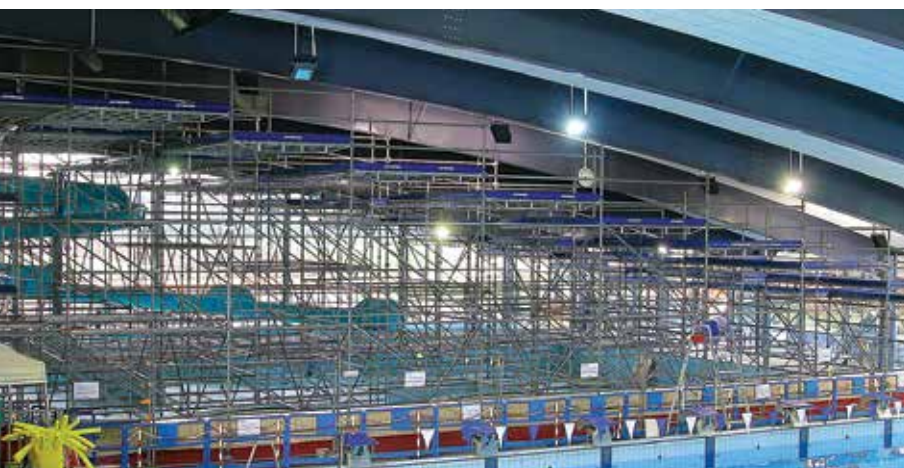
Montluçon: decks for the replacement of hangers in the swimming pool's false ceiling.
