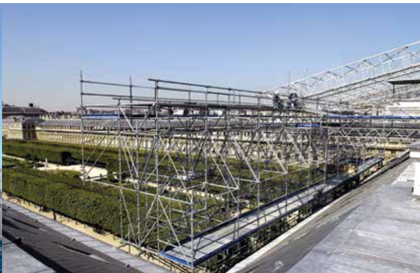
Paris, Palais Royal: temporary roof for renovation work to the headquarters of the Banque de France.
