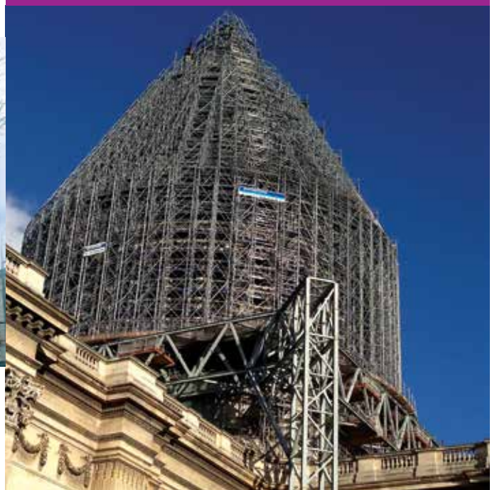
Paris, The Panthéon: 450 tonnes of scaffolding, standing free of the monument, for the restoration of the skylight, dome and drum.
