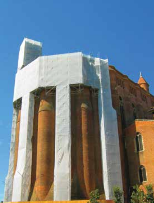
Albi cathedral: scaffolding for the restoration of the coping and stained glass.
