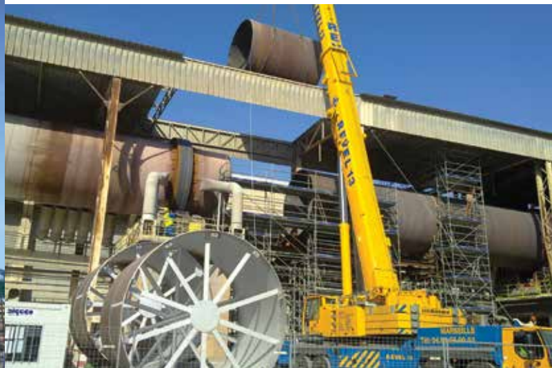
Ciments Lafarge: scaffolding and shoring for the replacement of a furnace shell.
