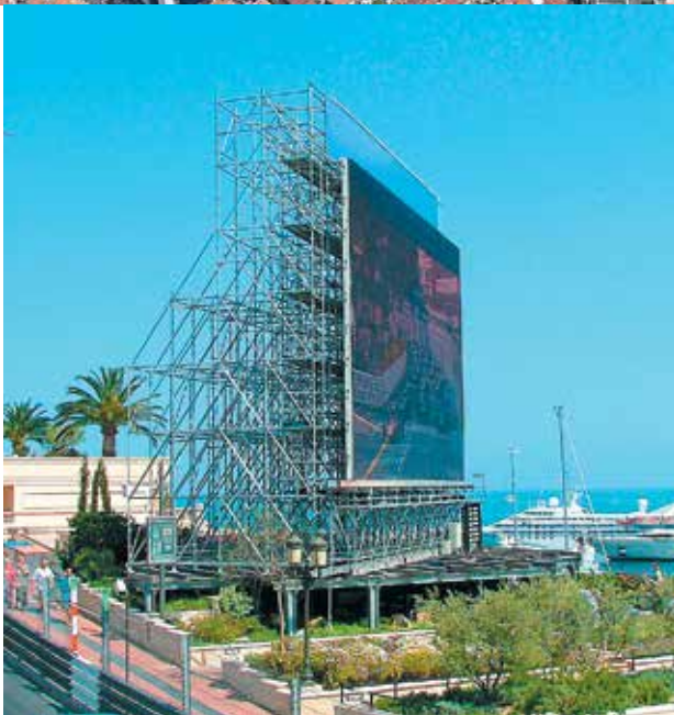
Monaco: for the F1 Grand Prix, spectator stands and related scaffolding such as walkways, access staircases and giant screen supports.
