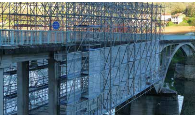
Arcambal bridge (46): mobile scaffolding for renovation works.
