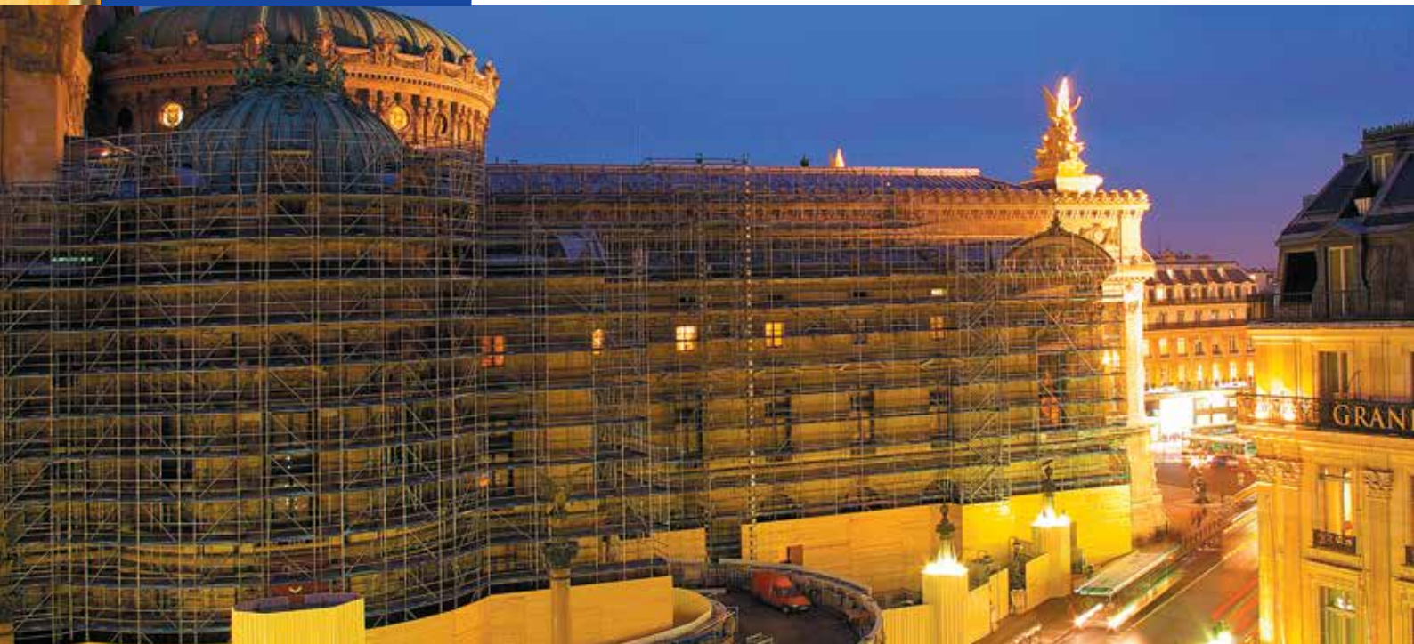
Paris, Opéra Garnier: scaffolding for the restoration of the west facade and cupola.
